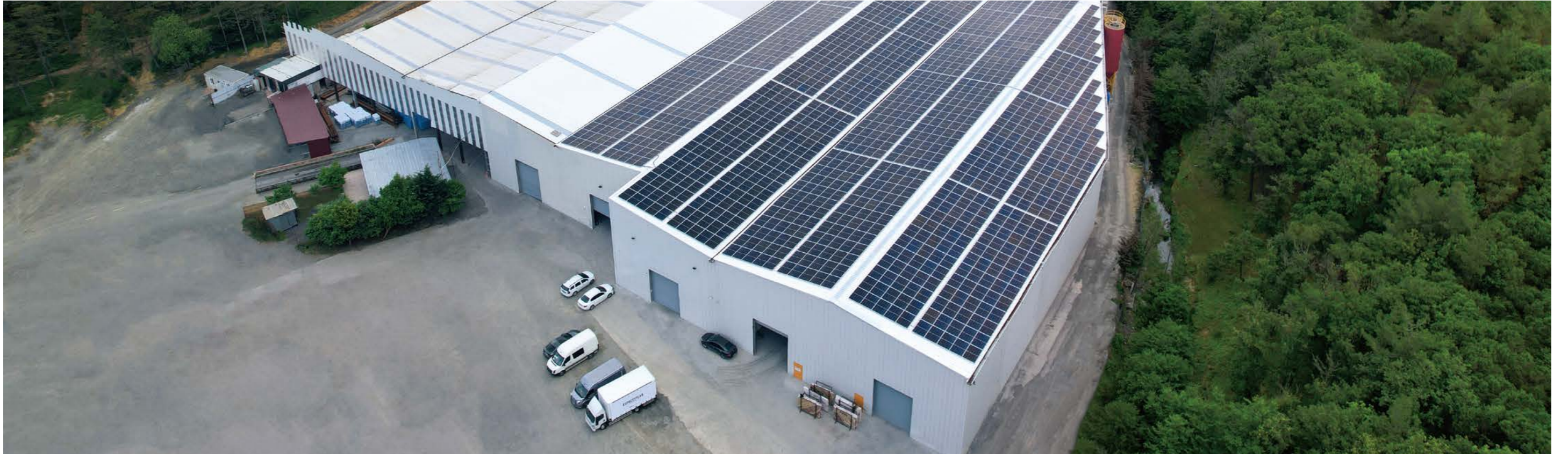
04 Energy Cost Reduction for Mineral Water Factory Turkey, 900kW KSG-120CL-M0
